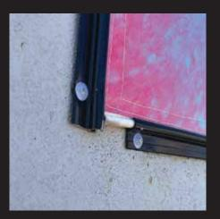
The Sail Track banner system is essentially a vinyl banner, manufactured with a high strength roped edge to allow installation into aluminium tracks to create a framed edge.
